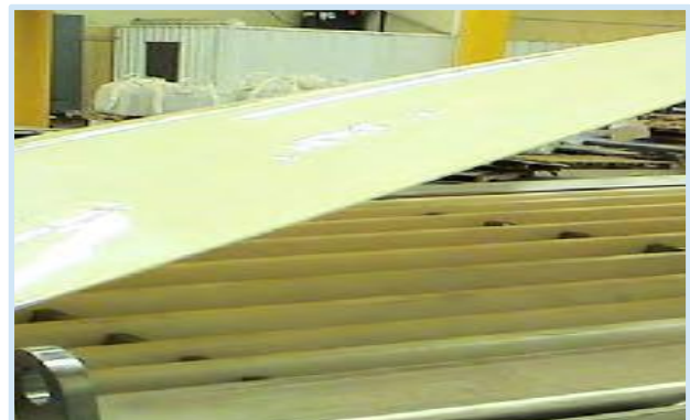
Belt repaired on site.
